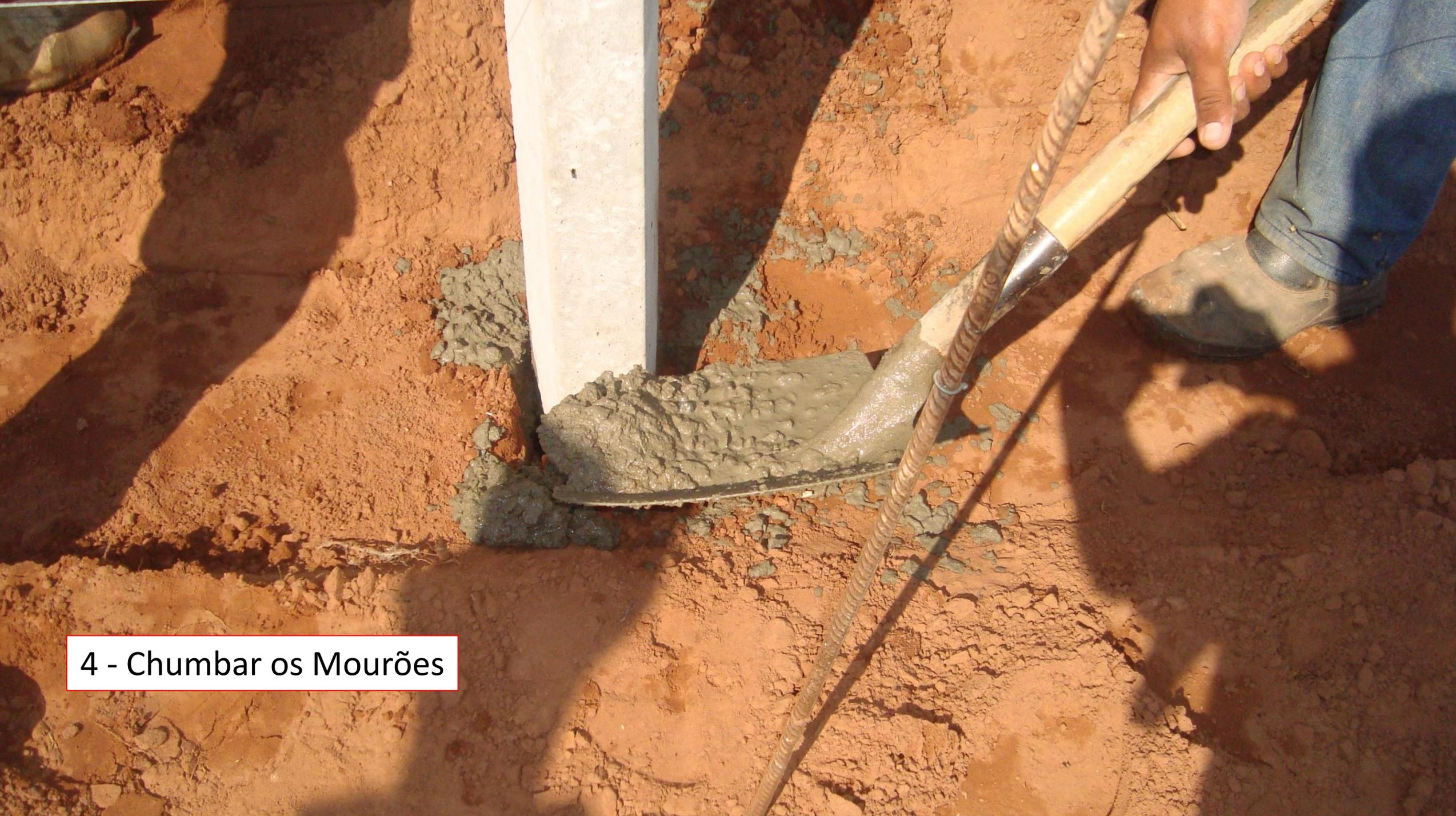
A close-up photograph of a construction worker's hands using a rebar to level concrete in a trench. The worker is wearing blue jeans and a black safety boot. The rebar is being held against a white formwork on the left side of the trench. The concrete is a light grey color and is being smoothed out. The surrounding soil is reddish-brown. The scene is brightly lit, casting shadows on the ground.
